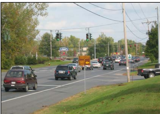
Figure 7: Signal and intersection spacing – As illustrated below, when signals are too close together the queues can spill back and block neighboring intersections.
