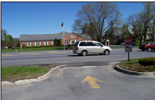
Figure 4: Driveway Channelization - As Illustrated Below, Prevents Left-Turning Traffic from Accessing the Primary Roadway
