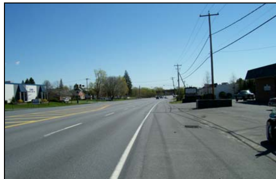
Figure 3: Frontage Road Installation - The image on the left illustrates use of a frontage road. Frontage roads allow for a single intersection on the primary road while providing direct access to individual parcels. In the absence of a frontage road a primary road can suffer from frequent and wide curb cuts as illustrated in the image on the right.
